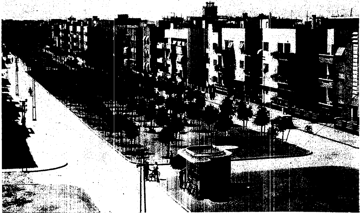
Rothschild Blvd. during the late thirties - a homogeneous succession of isolated buildings
