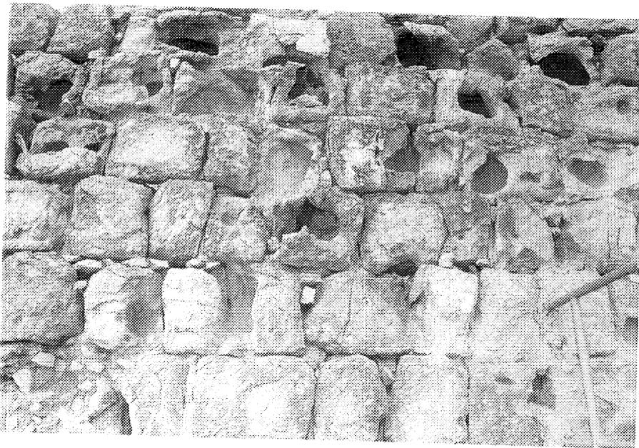
Eroded soft lime stone
