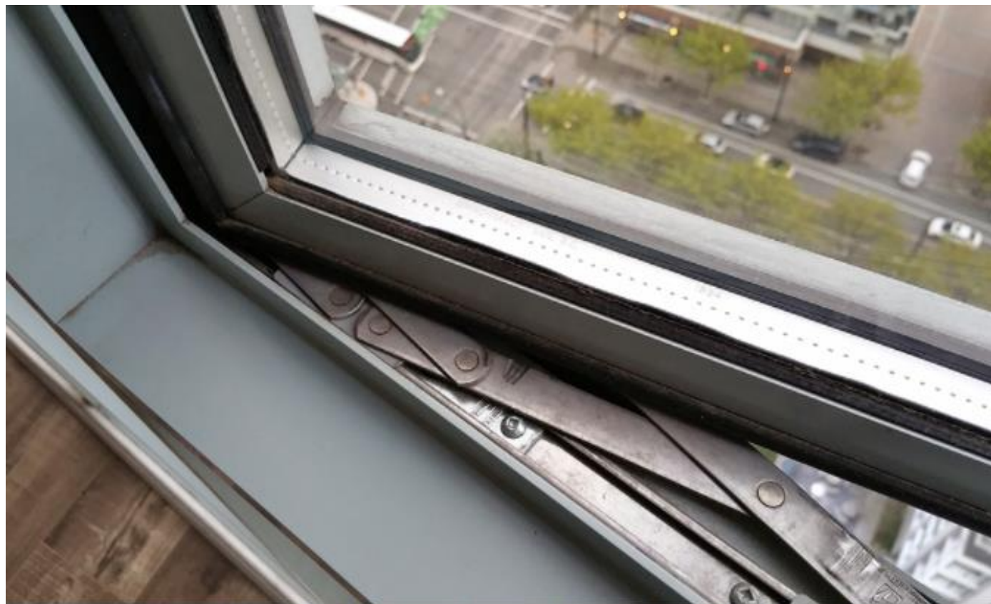
A close up of the stoppers we had installed to restrict our windows to opening only about 4 inches.
