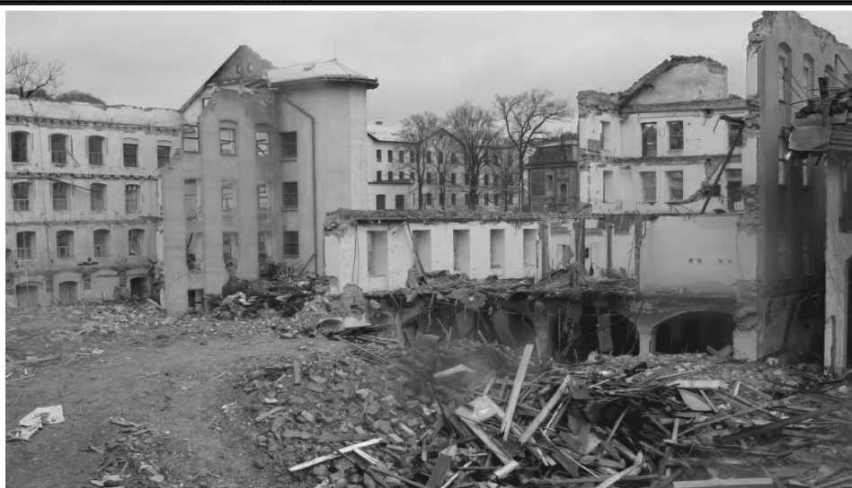
The lower part of the Schindler factory next to a demolished 19th-century building. (photo credit: Eva Munk/JTA)
