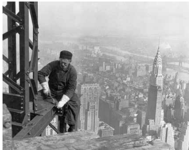
Lewis Hine, A Workman on the Framework of the Empire State Building (Old timer structural worker; Keeping up with the boys), 1930.
