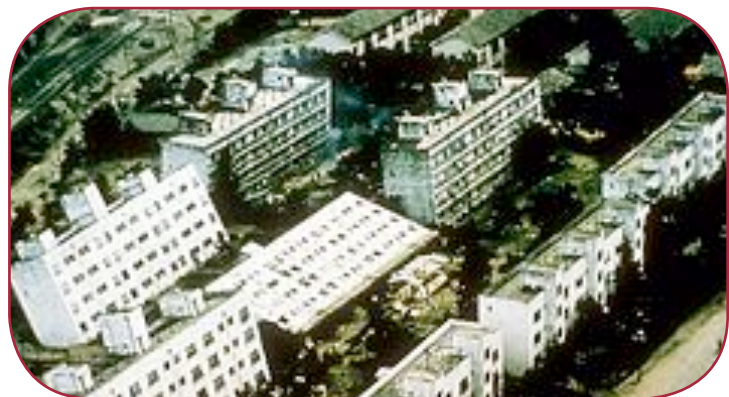
Liquefaction damage
