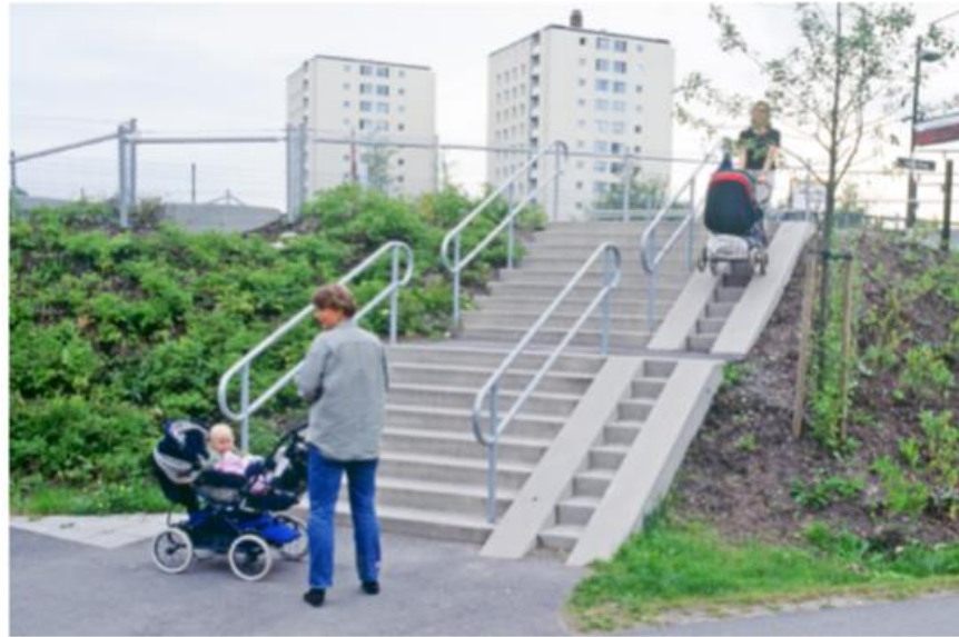
In Sweden, it is common to integrate ramps for bicycles and strollers into public staircases. This wheeling ramp makes accessing public parks and moving through the city easier, safer, and more convenient for families with children.
